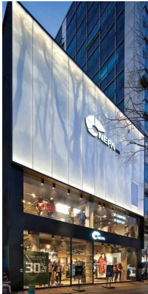
Fashion NEPA | Danpal® Single Facade System 16mm Architect: Mark Fran / de plus
