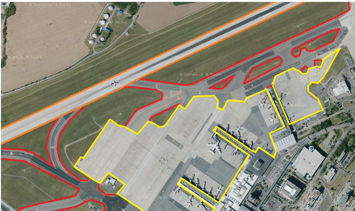
Figure 2.1. Václav Havel Airport Prague 1 , runways - orange, taxiways - red, aprons - yellow
