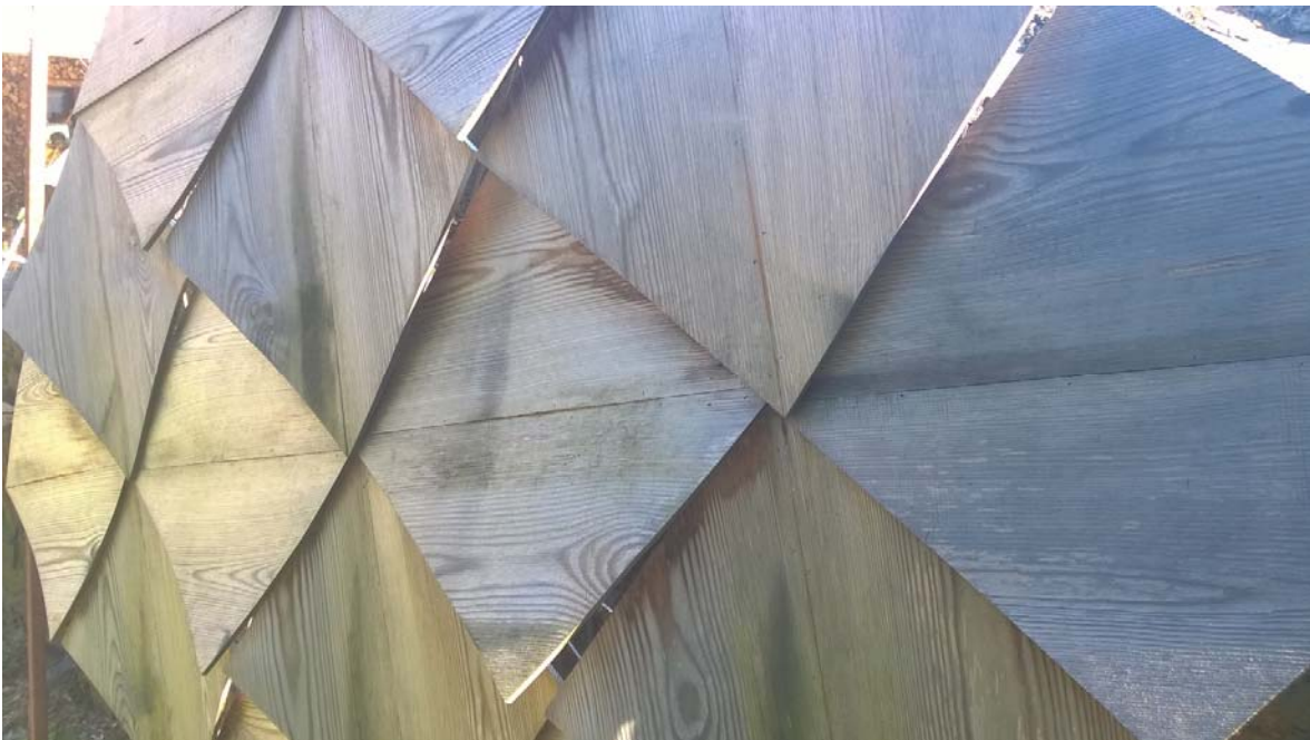
Figure 10: Ray 2 Prototype Being in Time-Based Co-Design with its Micro-Climatic Conditions and Blue Stain Fungi, Algae and Lichen that Inhabit It, All Regulating the Moisture Content of Wood, Thus Causing Warping. Notice Also the Organisation of Algae Habitation Caused by Material's Fibre Direction and Thus Moisture Distribution (photo: Davidová 2016)
