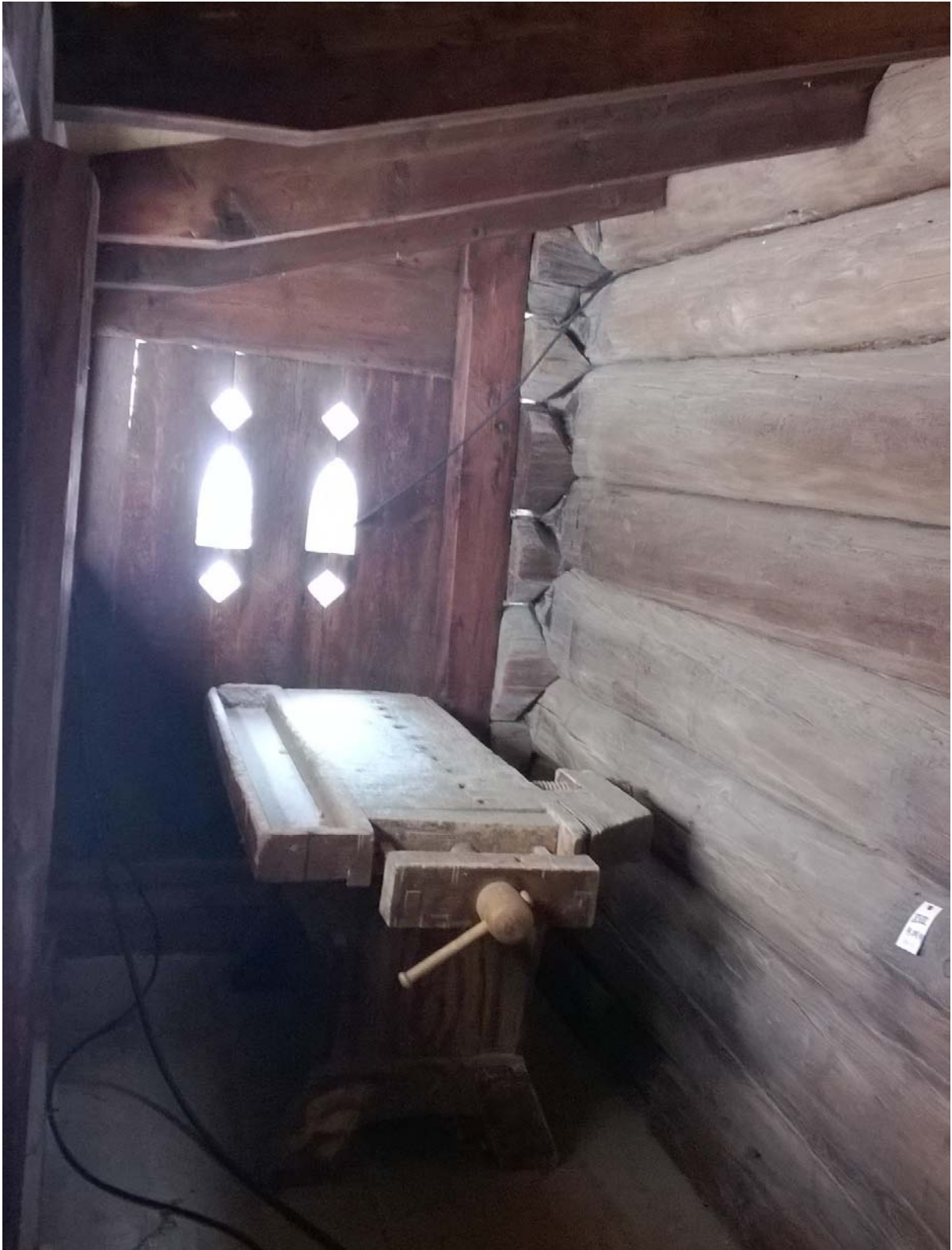
Figure 27: Svalgang of Hjeltarstua from 1763, recently placed in the Maihaugen Open Air Museum in Lillehammer (photo: Davidová 2016) shows the opportunity of indoor-outdoor environment including the range from social to climatic interaction while working actively.
