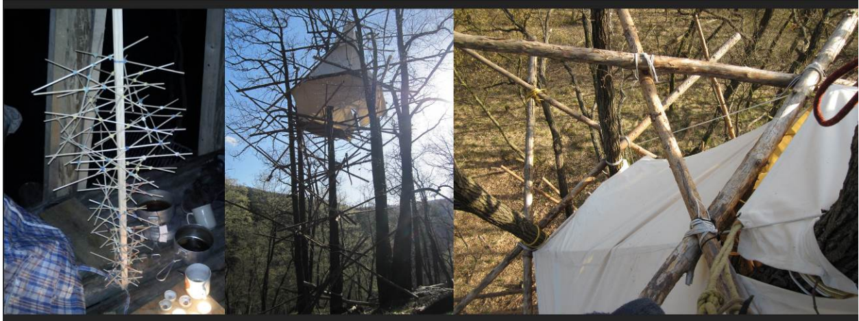
Figure 45: Davidová & Závada: SpiralTreeHouse – Project Start in 2010 (photos: Davidová 2010 and 2012)
