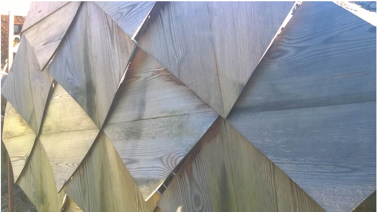
Figure 50: Ray 2 Prototype Being in Time-Based Co-Design with its Micro-Climatic Conditions and Blue Stain Fungi, Algae and Lichen that Inhabit It, All Regulating the Moisture Content of Wood, Thus Causing Warping. Notice Also the Organisation of Algae Habitation Caused by Material's Fibre Direction and Thus Moisture Distribution (photo: Davidová 2016)
