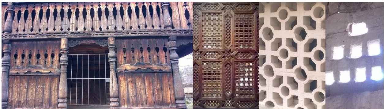
Figure 116: 'Breathing Walls' in Vernacular Architecture; from left to right: a) Norwegian Svalgang Screen of Loft from 1797, Oslo Open Air Museum, Norway (photo: Davidová 2016); b) Moroccan Mashrabīya from around 15 th Century, Houston Museum of Fine Art, USA (photo: Davidová 2016); c) Traditional South Portugal Screen Wall in Fishermen's Village Salema, Portugal (photo: Davidová 2016); d) Çavuşin Monastery from 964/5, Cappadocia, Turkey (photo: Davidová 2016)
