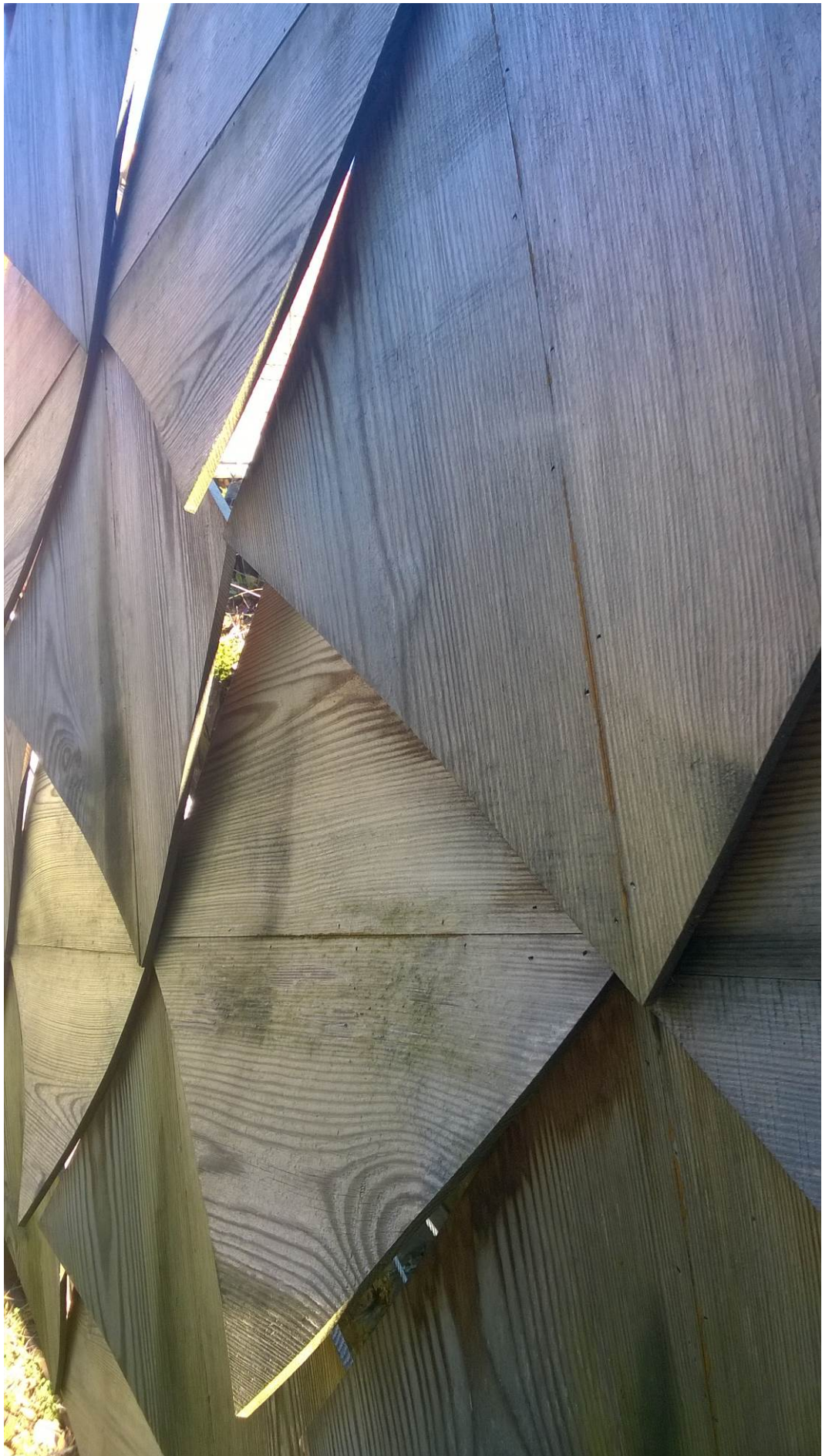
Figure 93: Prototype Ray 2 Performing after Three Years of Being Exposed to Climatic Conditions, Detail (photo: Davidová, 2016)
