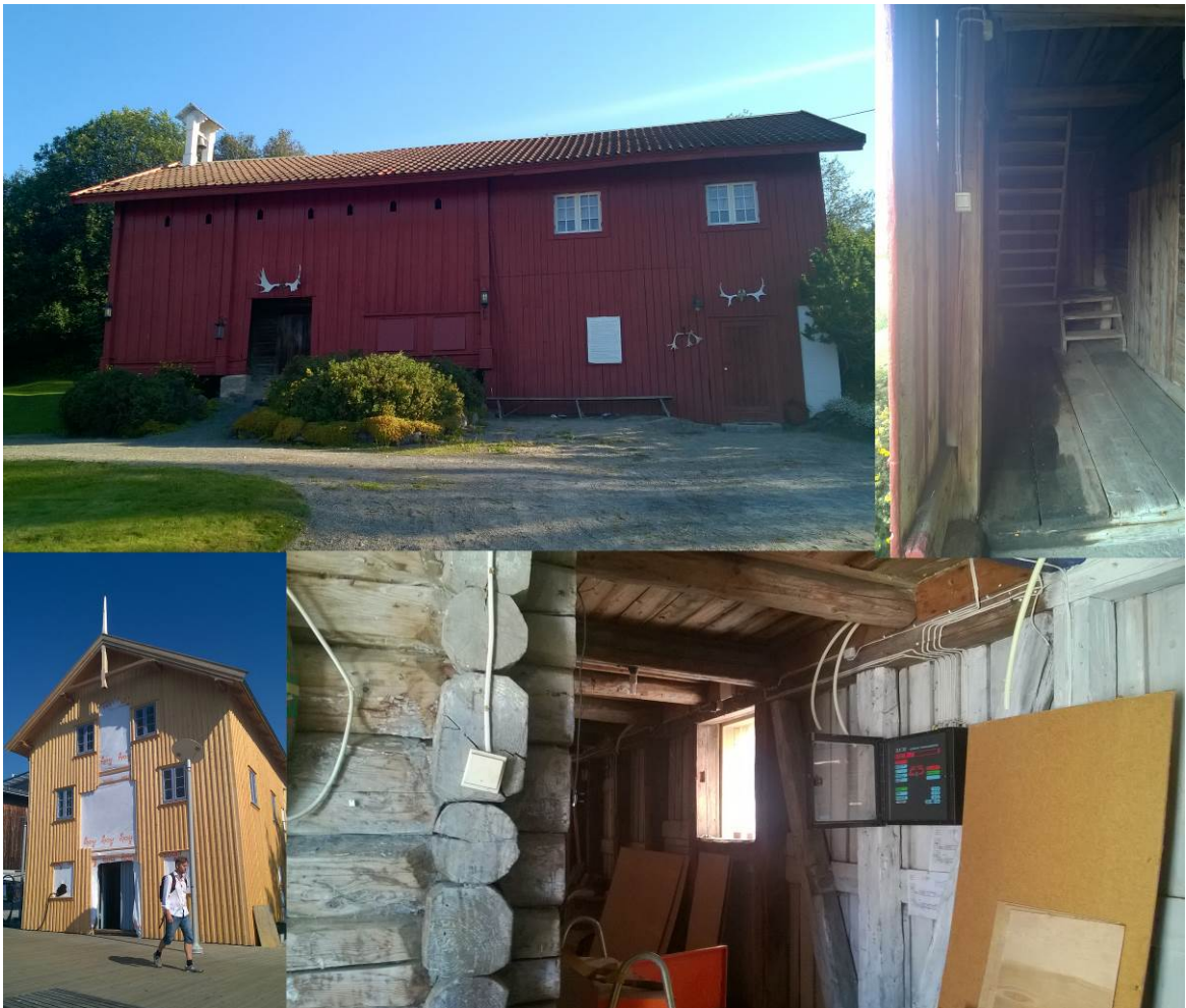
Figure 98: The Unclimatized Spaces, so called Onion System, in Norwegian Traditional Architecture (photo: Davidová 2015)
