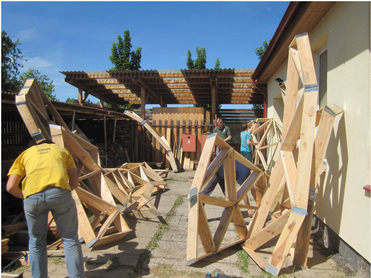
Figure 73: Ribs (photo: Davidová 2013)
