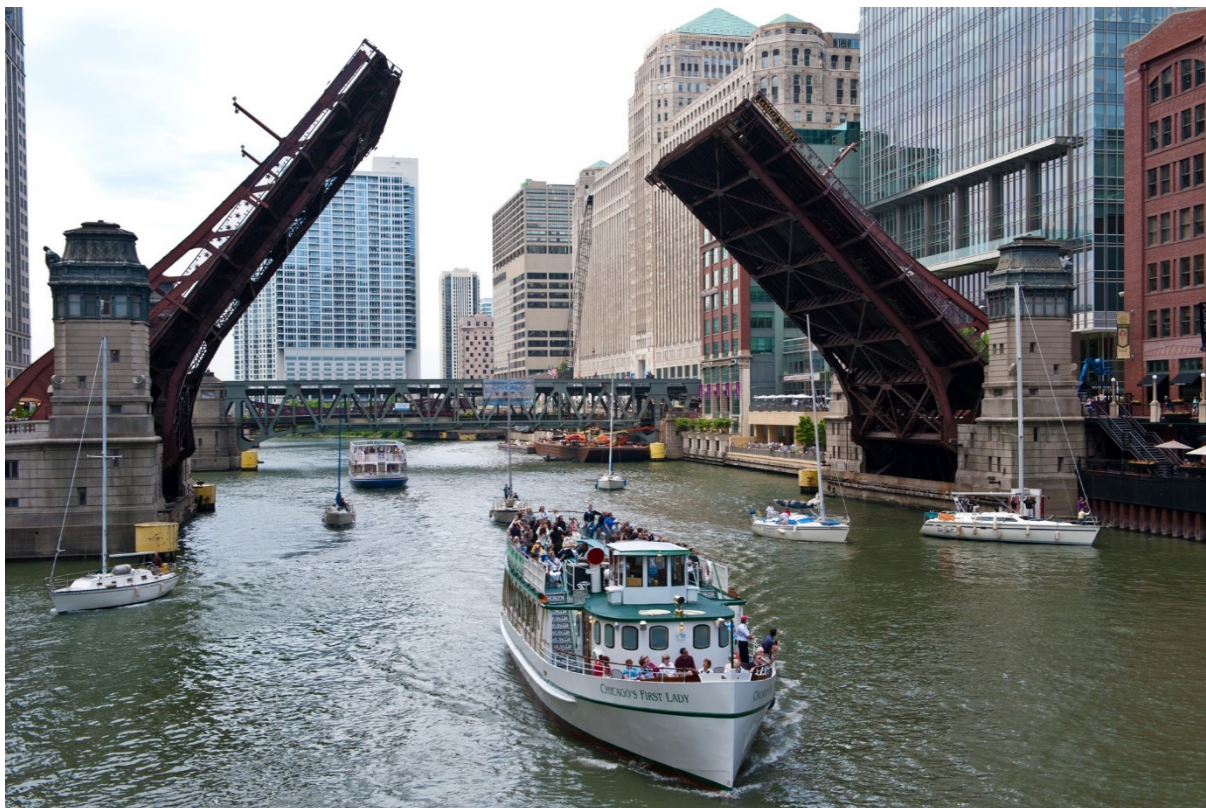
Obrázek 25 Downtown bascule bridge (Chicago, USA)
