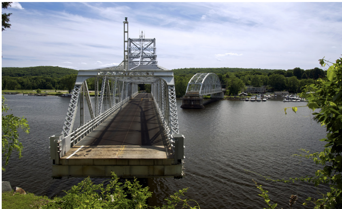
Obrázek 11 East Haddam swing bridge (East Haddam, Connecticut)
