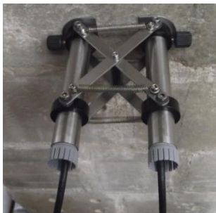
Figure 25 Ultrasonic test on the wall
