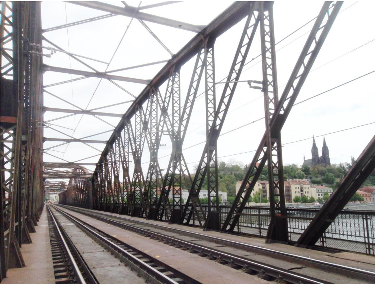
Figure 16. General view of the vertical elements and diagonals in the bridge.
