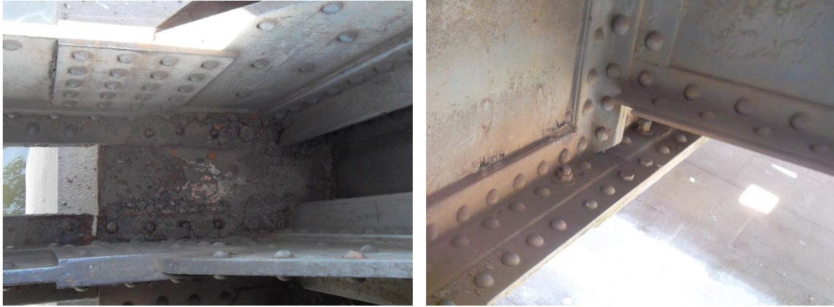
Figure 11. Bolts replacing rivets in different locations.
