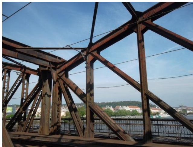
Figure 21. Typical connections in the railway bridge.
