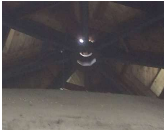
Figure 5 Roof ventilation hole
