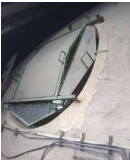
Figure 6 Fresco dome ventilation opening
