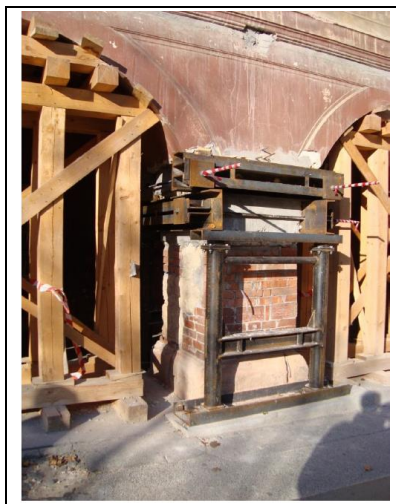
Figure 58: Steel Support for Lifting Building in Pohorelec 112, Praha [19]
