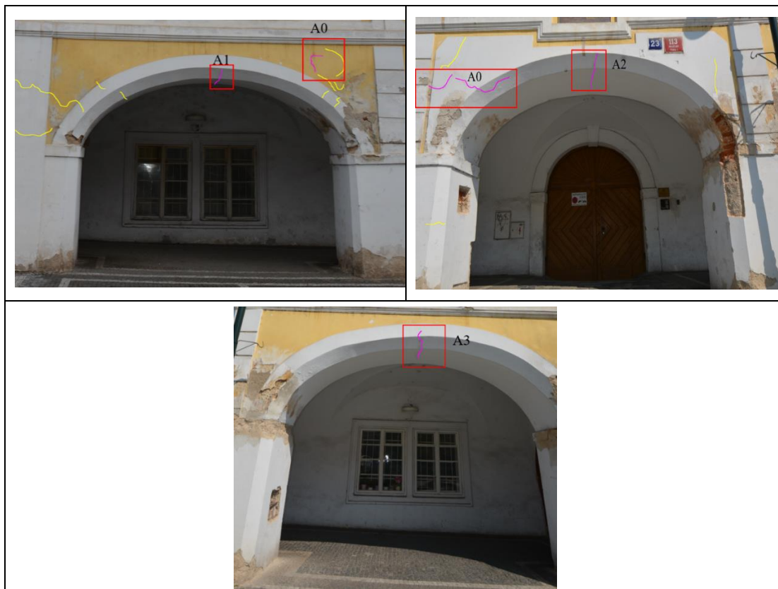
A1,2,3: Cracks on Arches
