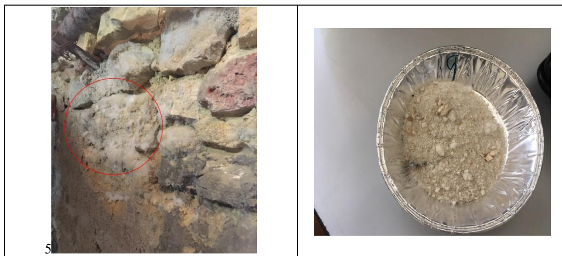
Figure 38: Salt Crystallization in-situ
