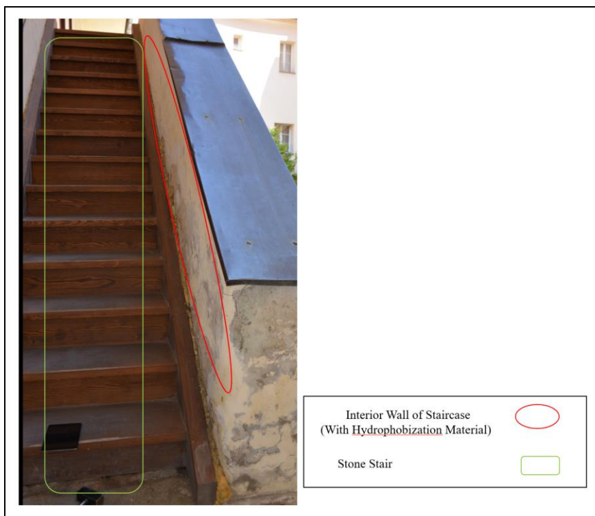
Figure 67: Detail Intervention for Interior wall of Staircase
