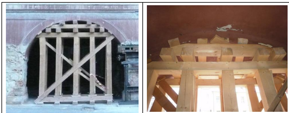
Figure 56: Wooden Support to Secure Structure of Building in Pohorelec 112, Praha [19]
