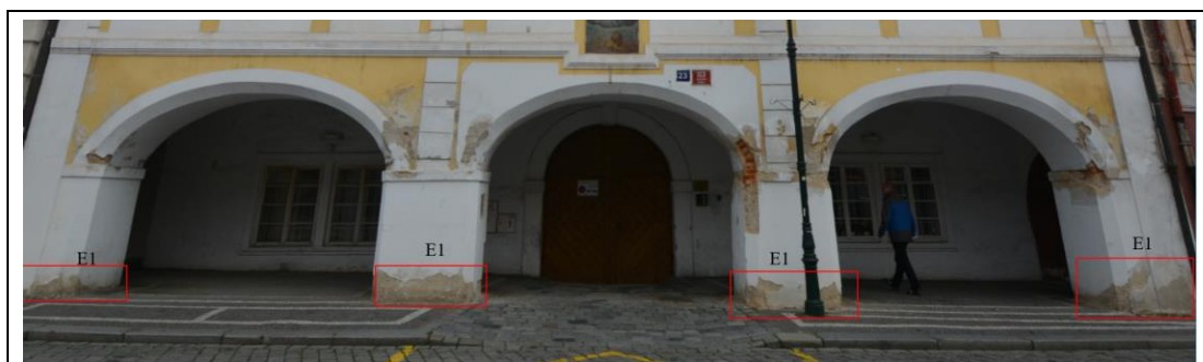
E1: Splashing Water and Rising Damp
