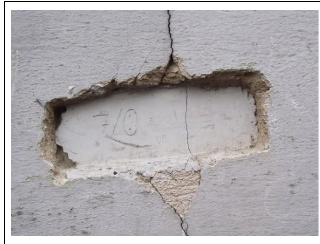
Figure 52: Plaster Placement in Masonry [2]
