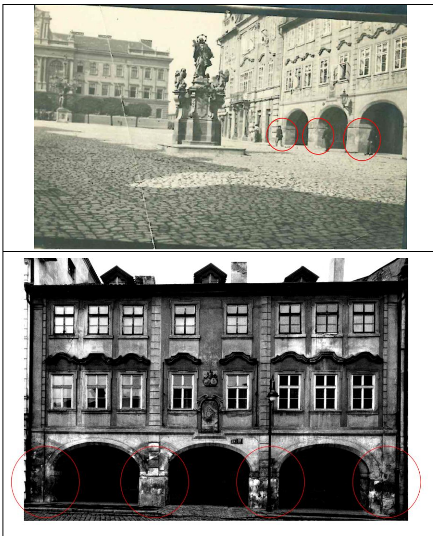
Figure 3: Building Strahovská FARA in 20 th Century (Strahov Monastery Provided)
