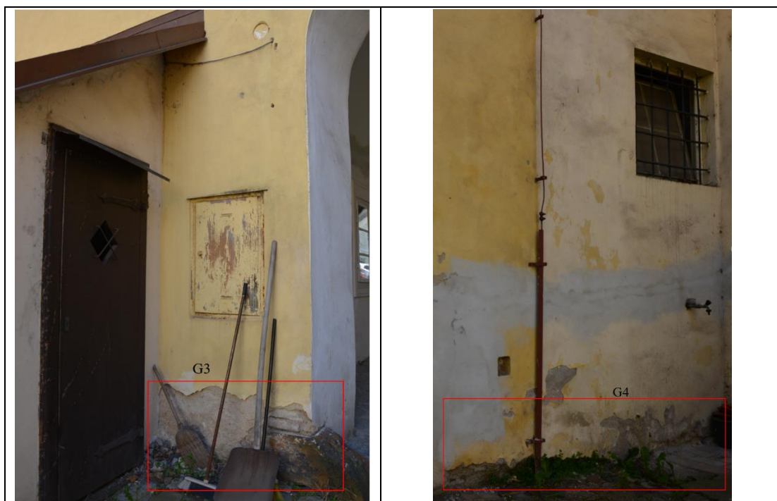
G3; G4 : Splashing Water and Rising Damp
