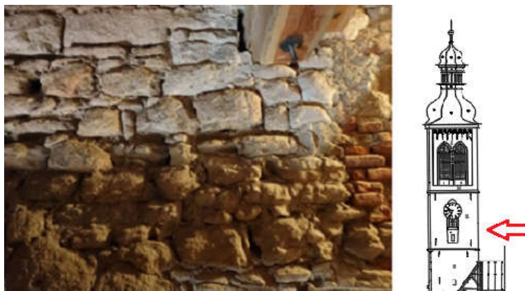
Figure 4 – Inside layer of the double leaves masonry wall
