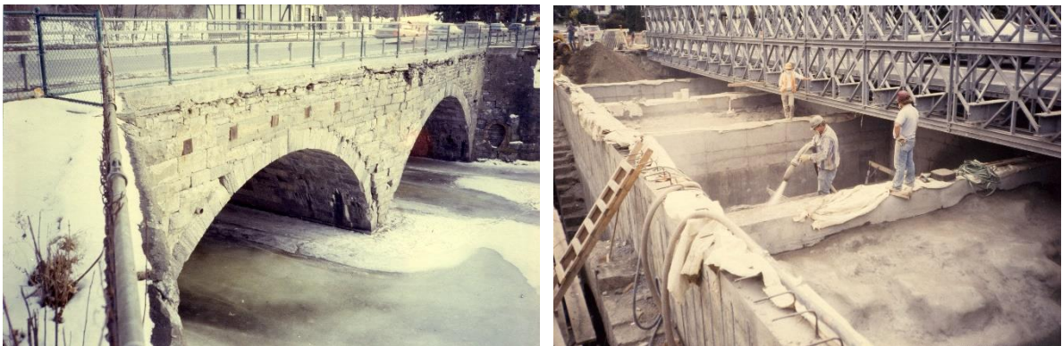
Figure 3 – Pawling Avenue bridge intervention, 1986
