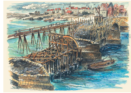
(b) Construction of the Charles Bridge
