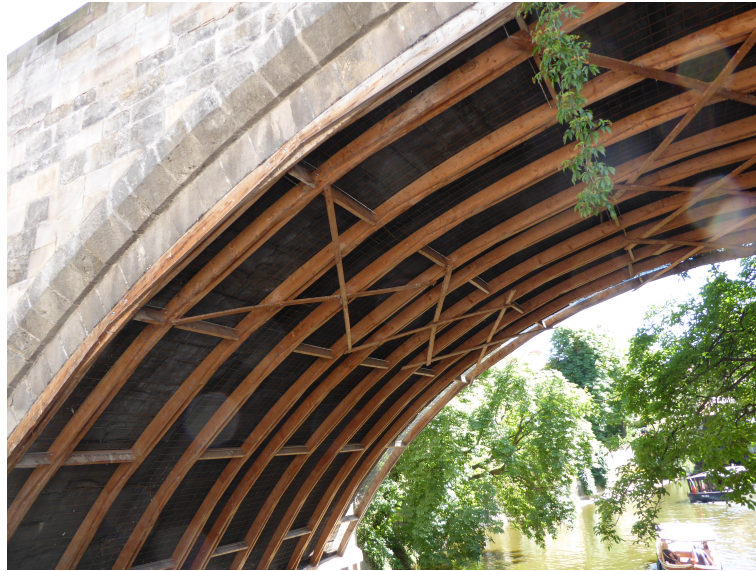
Figure 1.6: Current scaffolding on the 14th arch
