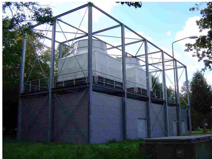
Figure 3-6 Cooling towers [23].
