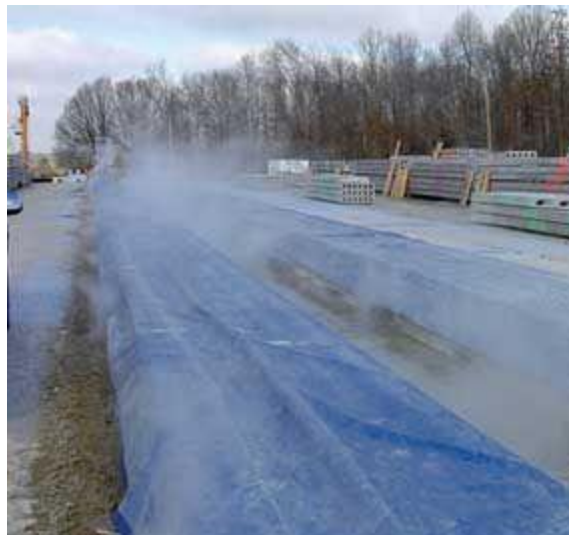
Figure 2-5 Steam curing of hollow-core slabs
