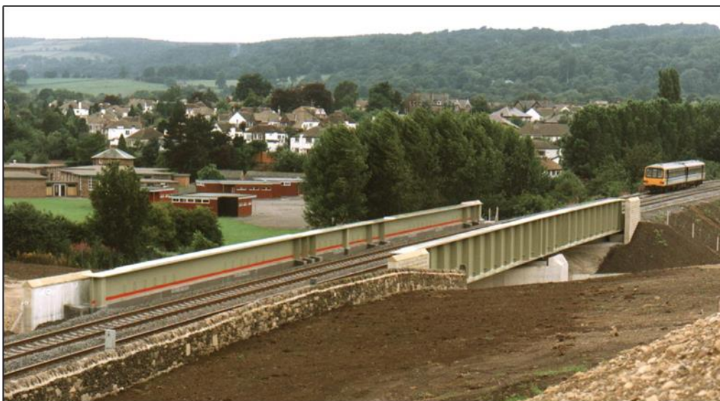
Figure 2: A Half-through Bridge [1]
