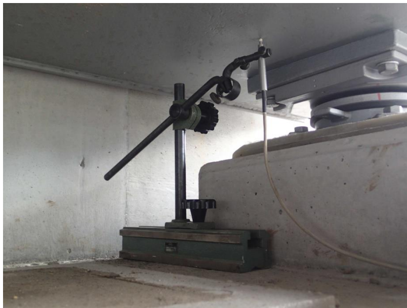
Figure 18: Inductive deflection sensors at the abutments
