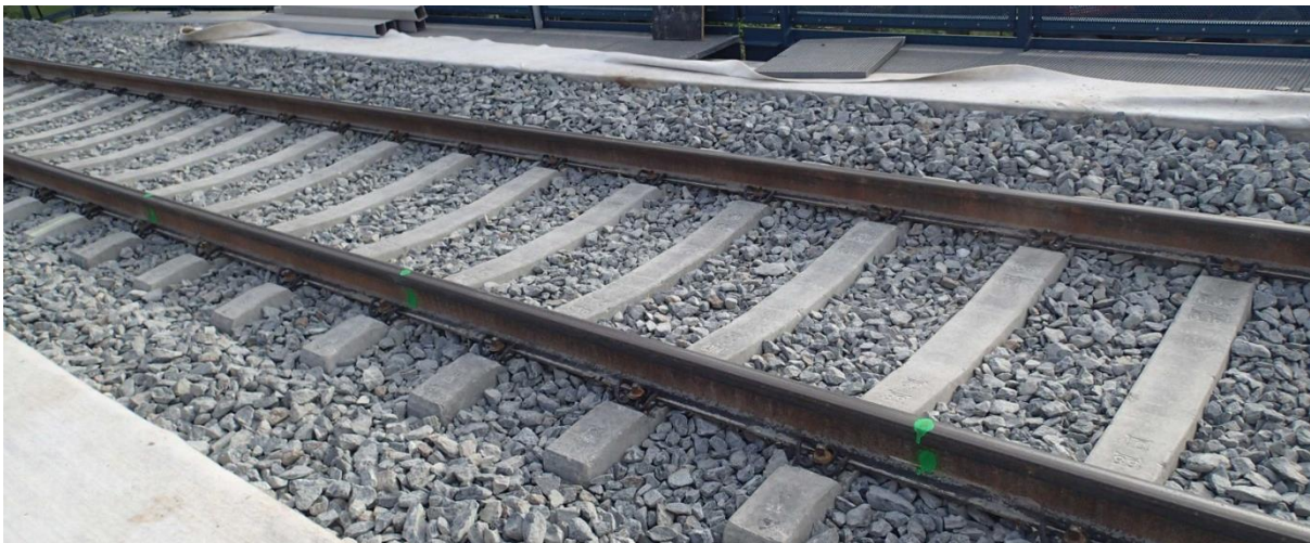
Figure 8: Railway track resting on ballast
