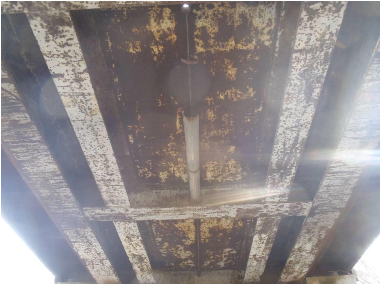
Figure 11: Top and bottom views of the old bridge
