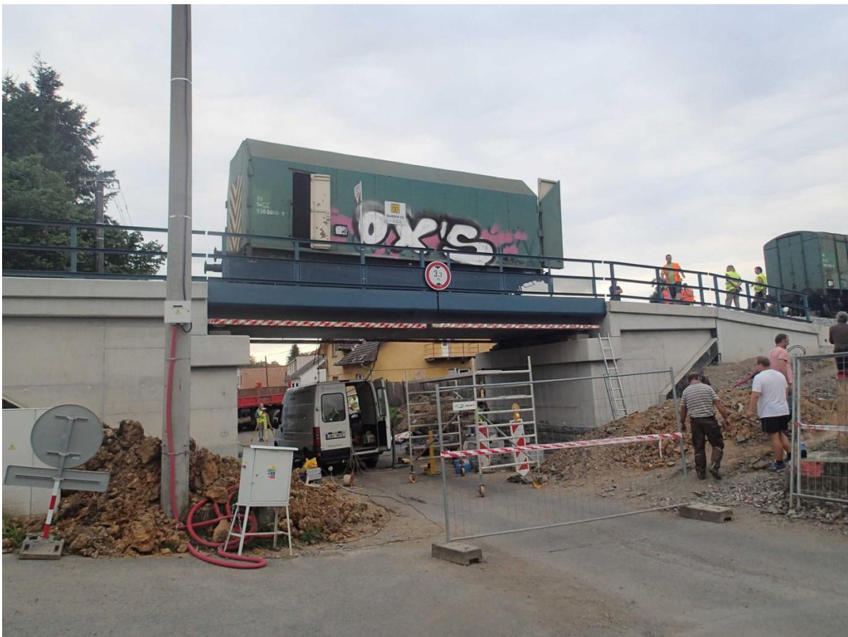
Figure 24: Wagon placed on the bridge for LC1
