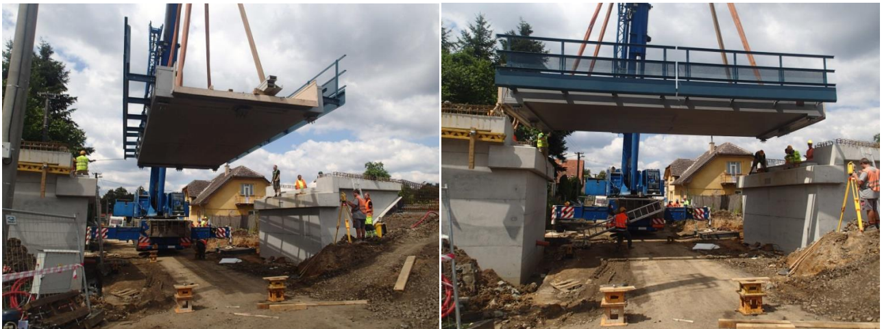
Figure 17: Erection of the bridge (On-site placement)
