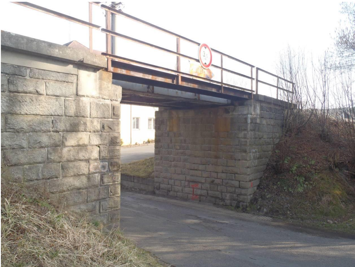
Figure 10: Side views of the old bridge
