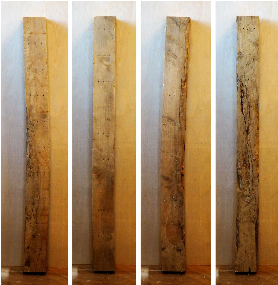
Photo 3–9 The Column S after the static load test
