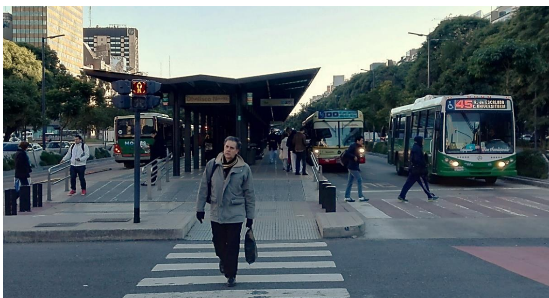
Fig. 20: Center station serving both directions; Stations located near intersections due to block length
