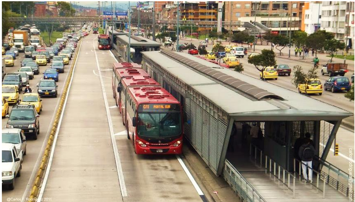
Fig. 3: TransMilenio in Bogota – median busways with passing lanes at stations (9)
