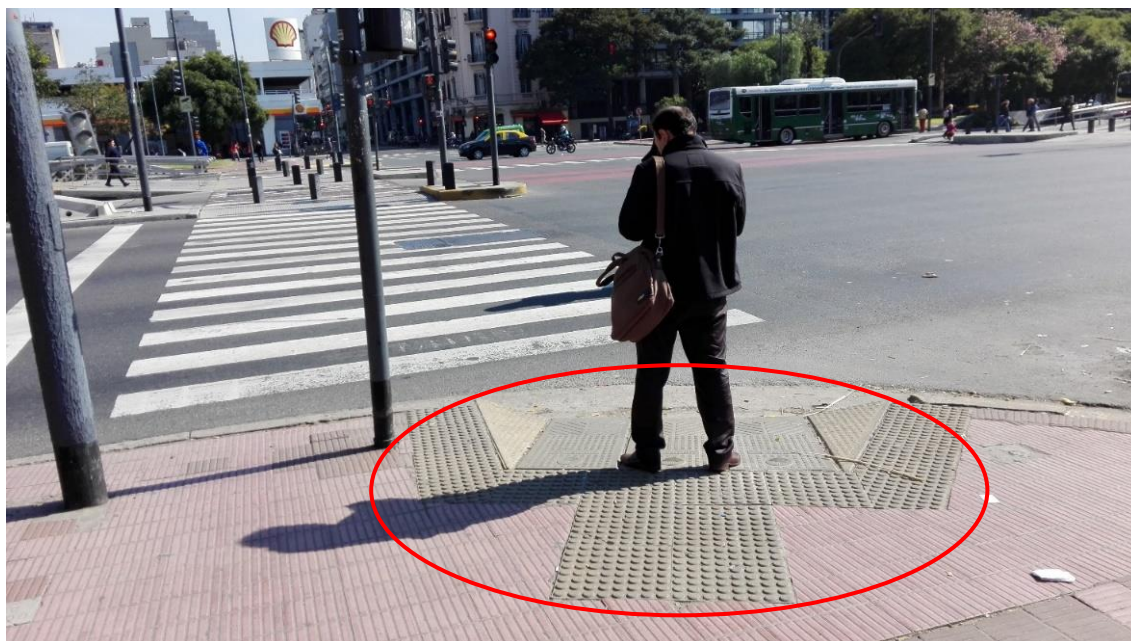
Fig. 31: Direction of the back edge and rows of blister is not in the direction of the crossing
