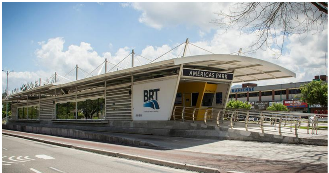
Fig. 52: Station of BRT Transcarioca (54)
