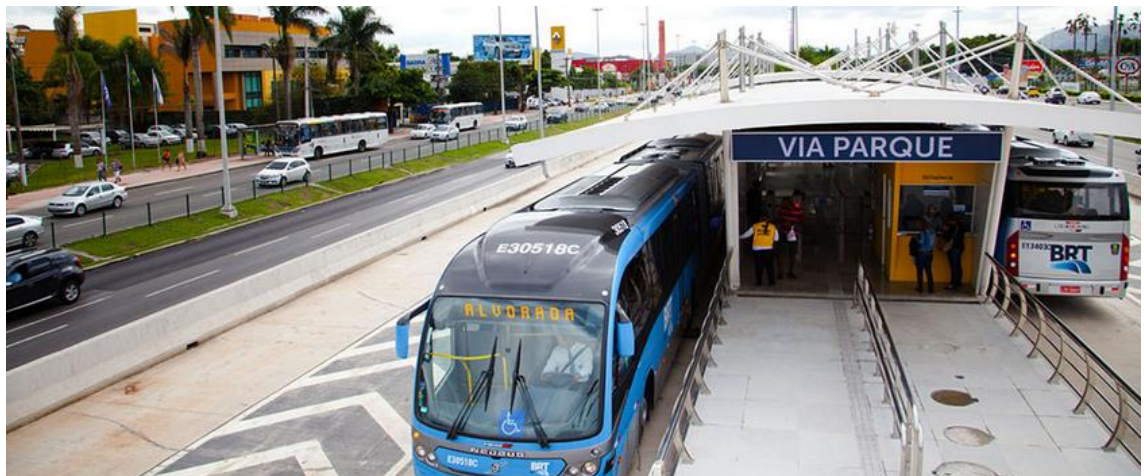
Fig. 51: Center station serving both directions, Passing lanes at the stations (59)
