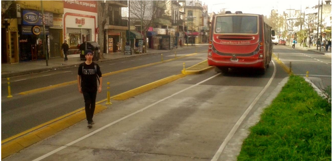
Fig. 44: Pedestrians entering the busway to enter the station
