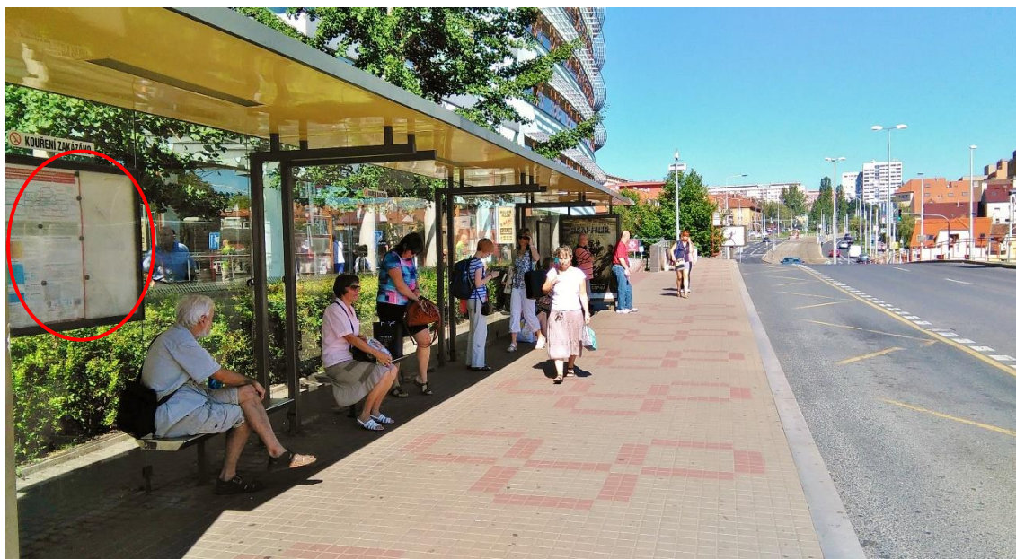
Fig. 61: Stop with a bigger shelter partly weather – protected; on the left side of the picture there is static passenger information
