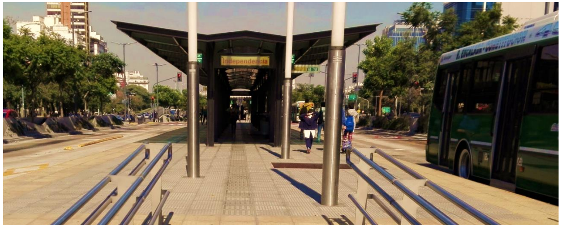
Fig. 21: Station of Metrobus 9 de Julio; Total width of the stations is 8 meters and internal width 2 meters
