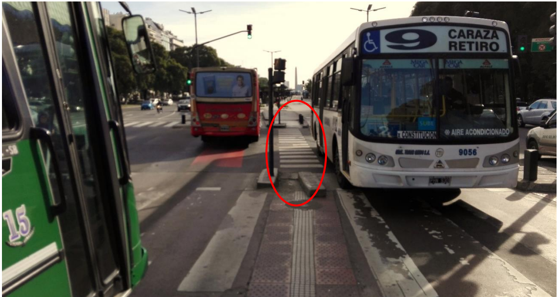
Fig. 26: Narrow dangerous pedestrian crossing between two busways
