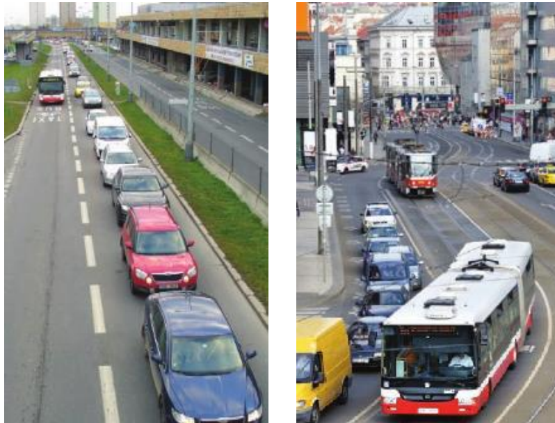
Fig. 57: Dedicated bus lanes (Opatovská Street) and tram rail shared with buses (Plzeňská Street) (71)
