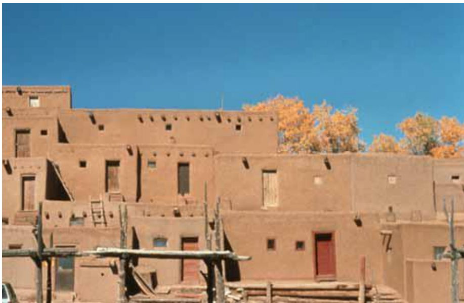
2.5 Adobe constructions in Pueblo de Taos [6].
