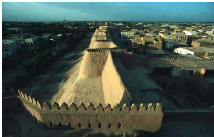
2.2. Walls of Itchan Kala [6].
