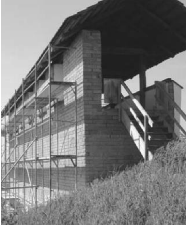
1.5. Reconstruction of mud-brick wall, Heuneburg, Germany, 6th century BC [2]
