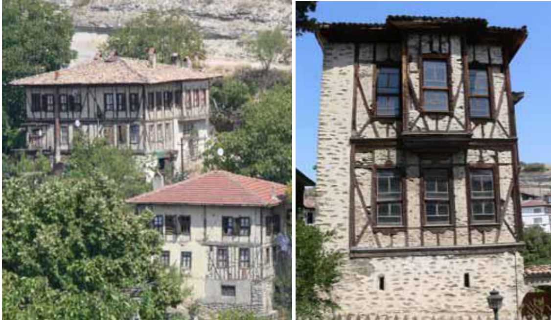
2.3 - 2.4 Wood-framed buildings in Safranbolu [6]
