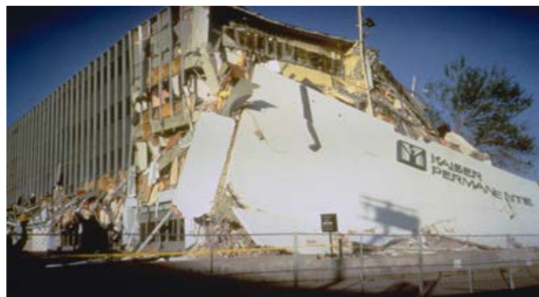
Figure 1. 3: Building collapsed during the earthquake as a result of LCF [3, 4]
