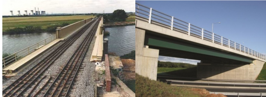
Figure 1. 9: Use of S275 and S355 steels in typical railway and highway bridges [8]
