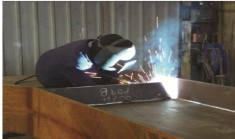
Figure 1. 8: Welding stiffeners onto a large fabricated beam [7]
