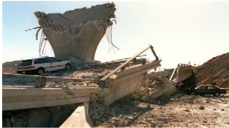
Figure 1. 4: Bridge collapsed during the earthquake as a result of LCF [3, 4]
