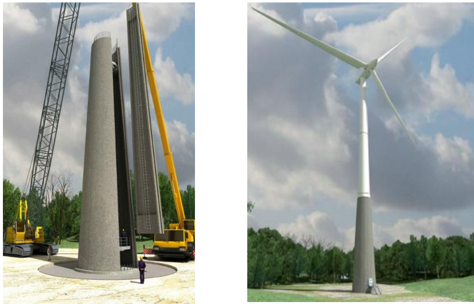
Figure 2.8: Crane assembling the precast concrete parts on left and on right side GRI hybrid concrete- steel wind tower ( www.gri.com )
