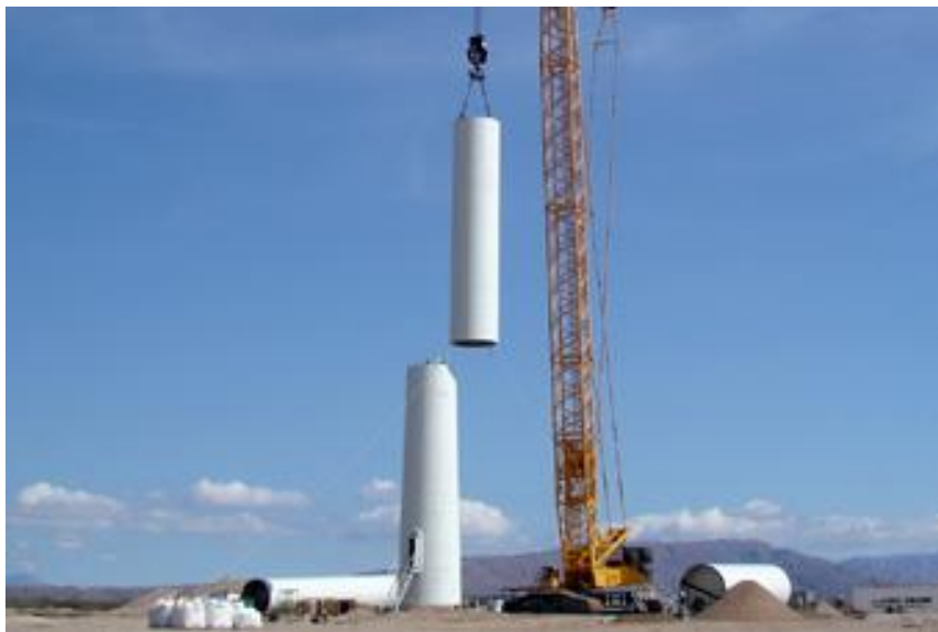
Figure 4.2: Conventional lifting procedure of tubular tower segments by Crane ( http://www.siemens.com )
