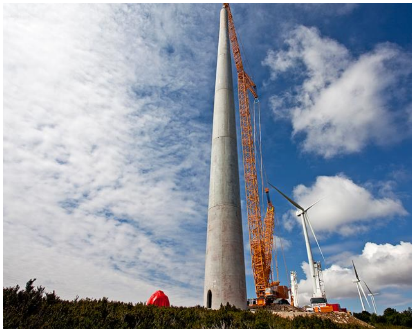
Figure 2.3: Concrete Tower for Wind Turbine ( www.acciona-windpower.com )
