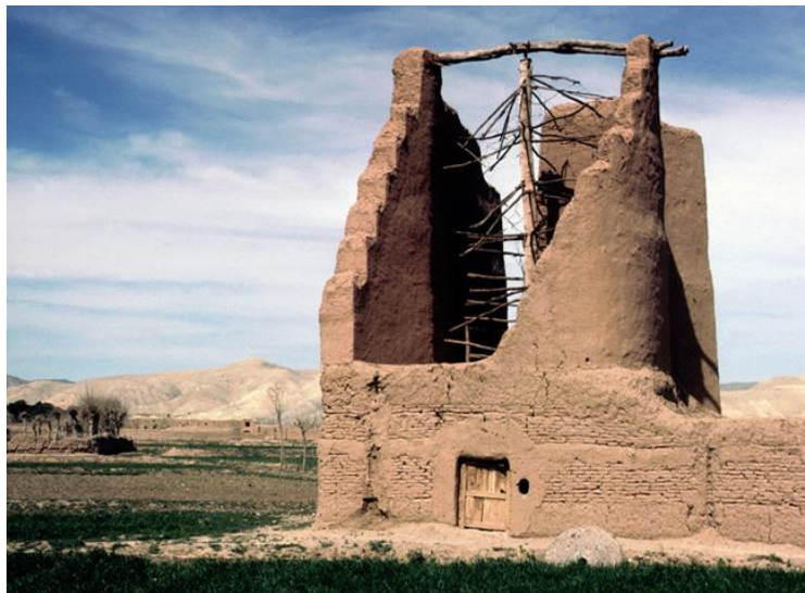
Figure 2.1: Afghan wind will with vertical axis (oratoryorphanage.org)
