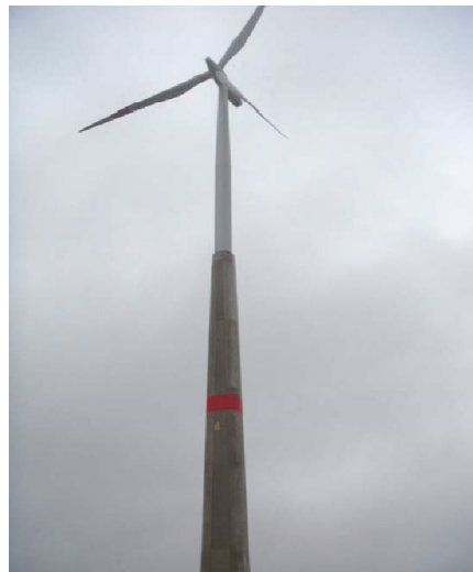
Figure 4. Concrete-steel hybrid tower
