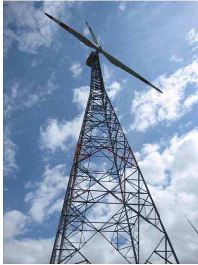
Figure 6. Steel lattice tower
