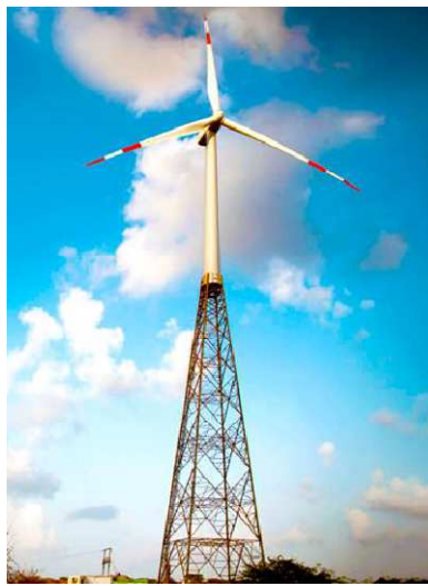
Figure 8. Steel hybrid lattice-tubular tower
