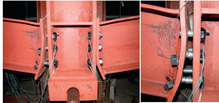
Figure 2.24. Failure mode of the flush end plate connection [28].
