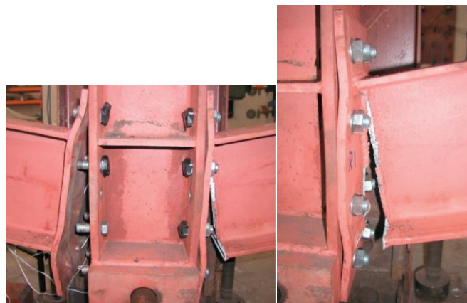
Figure 2.26. Failure mode of the extended end plate connection [28].
