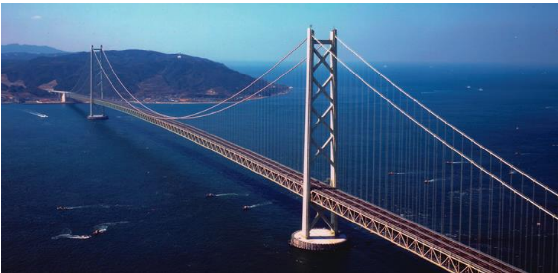
Obr. 5: Akashi Kaikyō Bridge (1991 m). [5]
