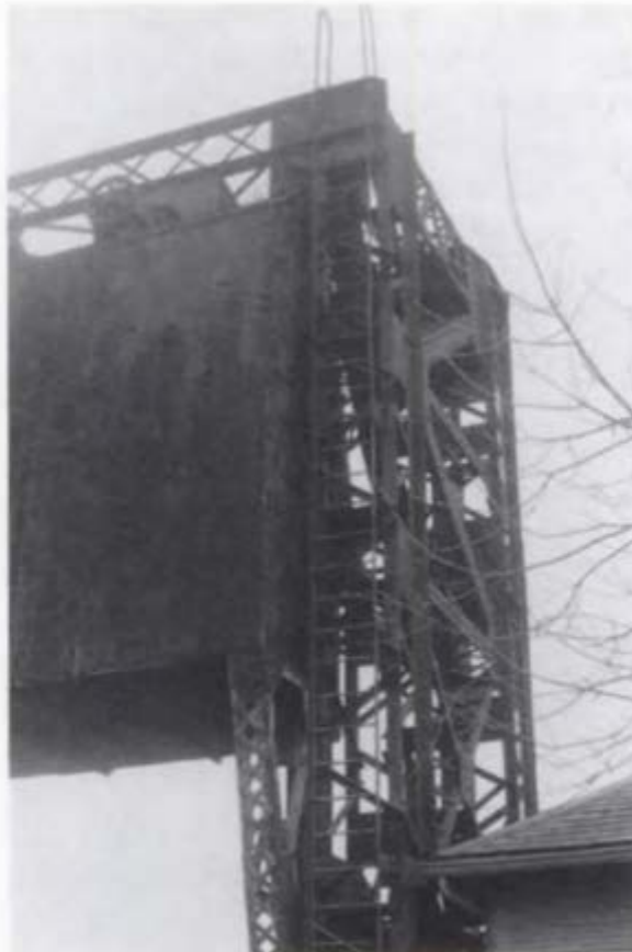
Figure 18-10 Chain Type Hand Drive. This bascule bridge is manually operated. The pulleys on top of the counterweight are fitted with chain loops, operated by persons on the ground, to raise and lower the bridge.
