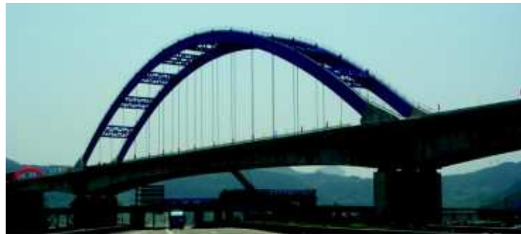
(a) Kunyang Bridge
