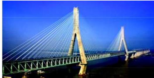
(a) Tianxingzhou Bridge
