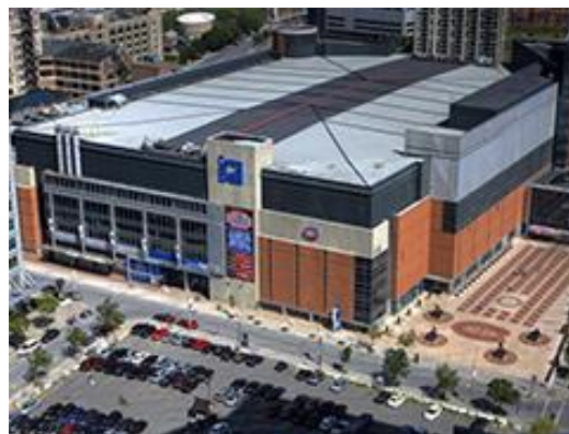
Obr. 11: Bell Centre Montreal [26]
