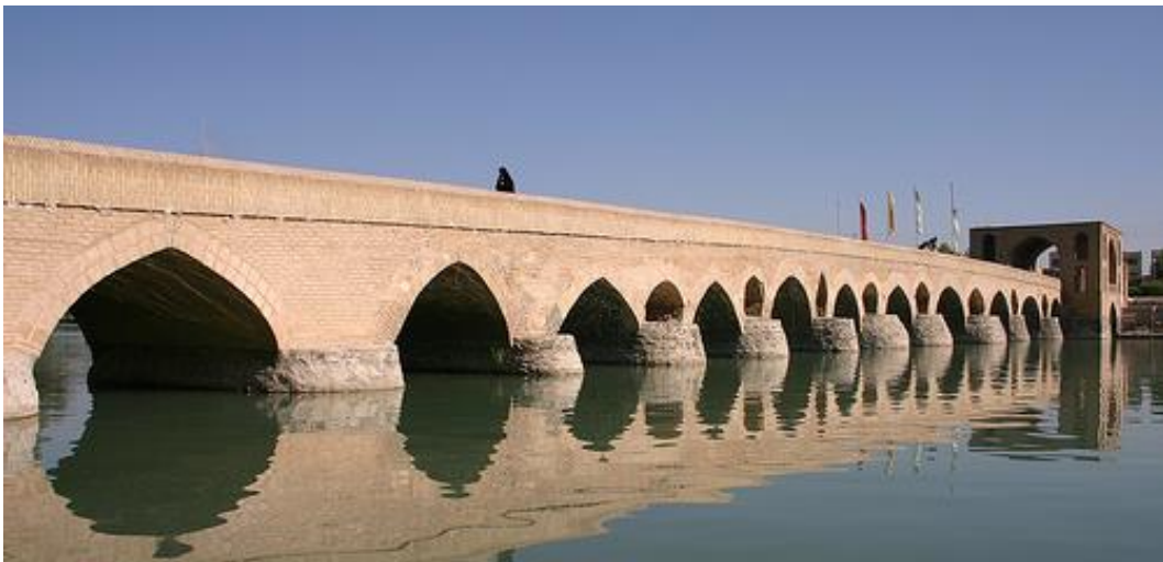
Obr. 1. 12 - Shahrestan bridge [xii]
