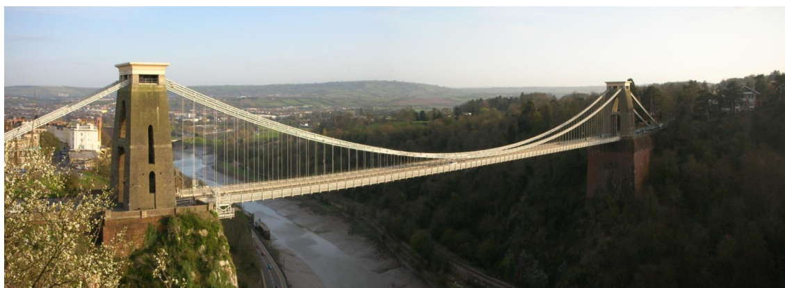
Obr. 1. 24 - Clifton Bridge [xxv]
