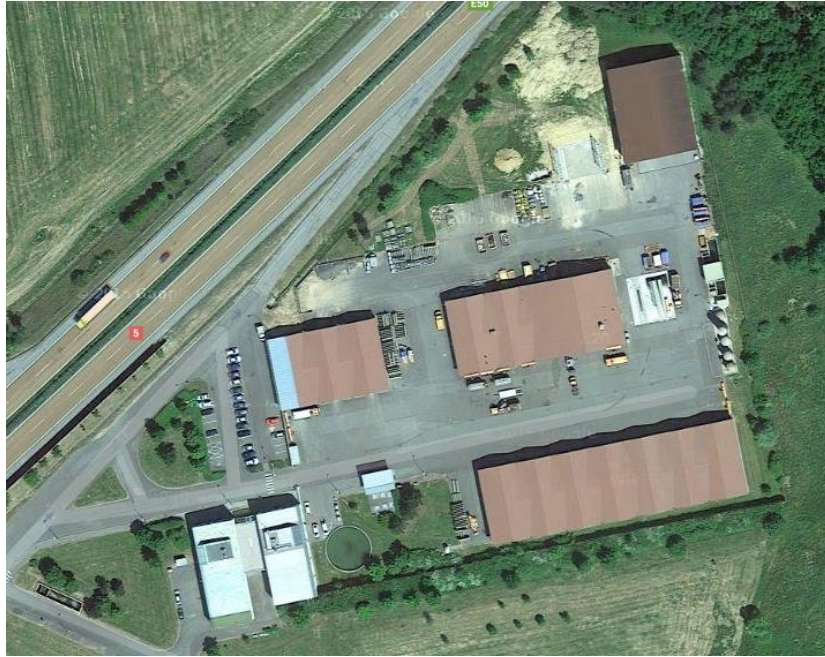
Fig. 20 - Highway maintenance center Svojkovice [48]
