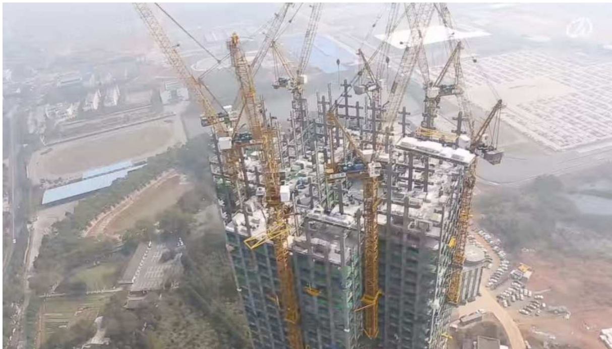
Figure 17 - Construction site of J57
