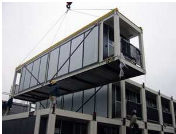
Figure 9 - Detailed assembling of the off-site units
