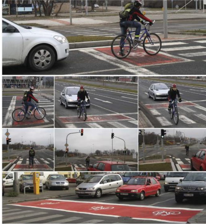
Figure 4.19: Bicycle box at intersection.
