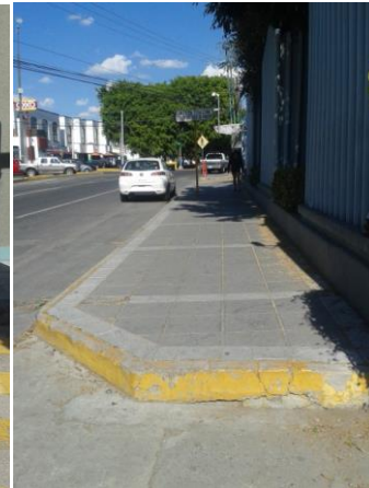
Figure 53: Step to the sidewalk
