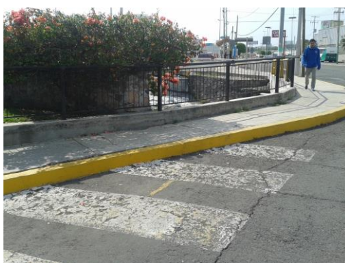
Figure 64: Sidewalk between the bus stop and the main entrance
