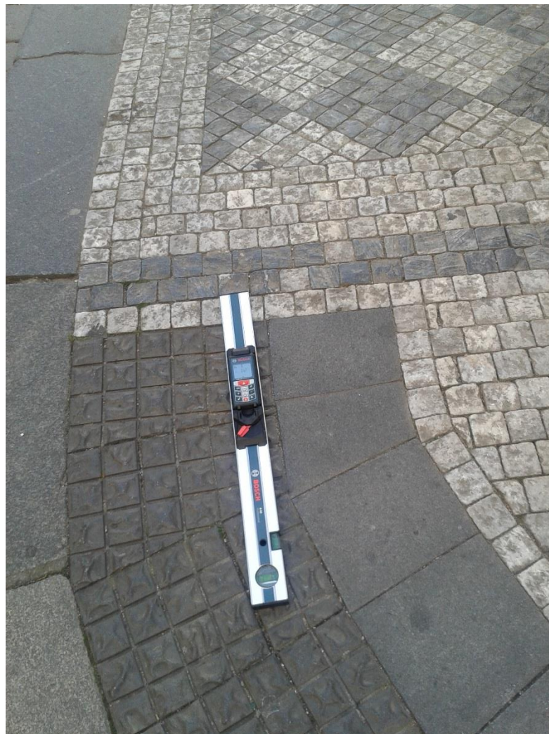
Figure 71: Cross slope on the pavement
