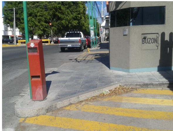
Figure 52: Step to the sidewalk
