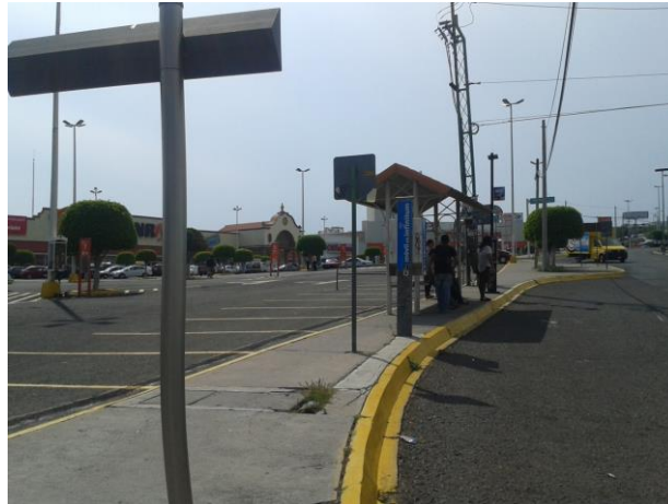
Figure 62: Bus stop on the street Ezequiel Montes
