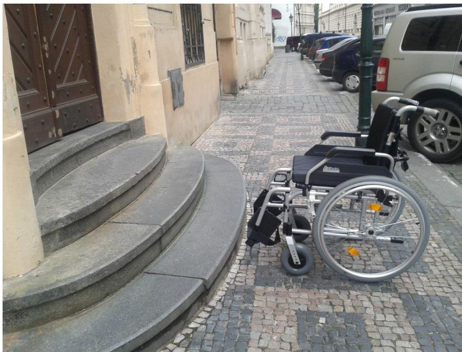
Figure 68: Entrance to the building on Kovniktská Street
