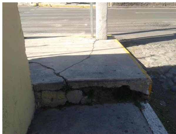
Figure 51: Same step to the sidewalk from the other side
