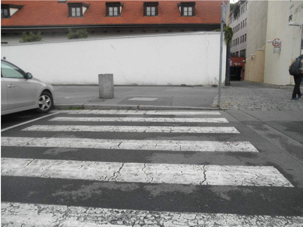
Figure 77: Crosswalk on the Na Florenci Street
