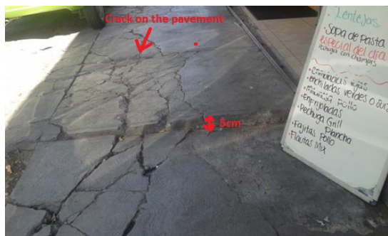
Figure 48: Main streets sidewalk
