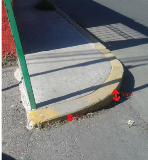
Figure 44: Other step to the sidewalk
