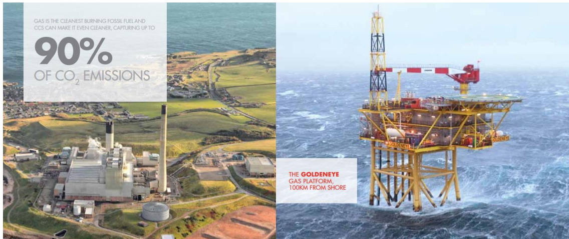
Figure 14: Peterhead Power Station on the left, Goldeneye gas platform on the right [25]
