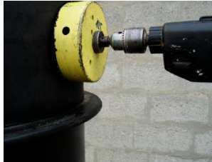
Drill the inlet borehole with a suitable crown drill
