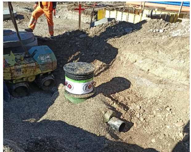
Picture 8: Burry of the reservoir with 4 – 16 mm
