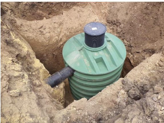
Picture 6: Installed tank
