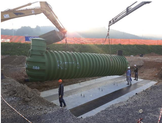
Picture 4: Installing the tank
