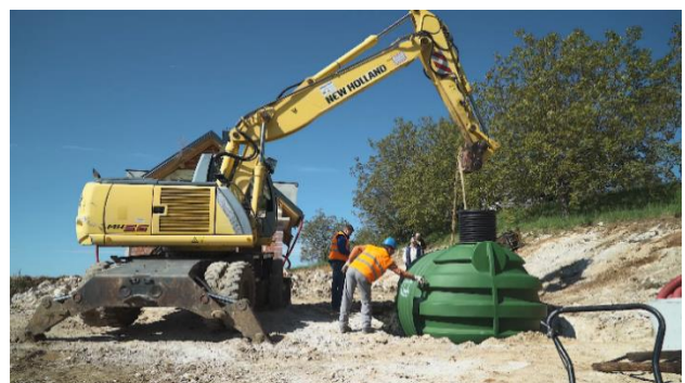
Picture 3: Installing the tank
