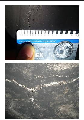
FIGURE 8. Flexural cracks with a width of 0.4–0.5 mm found on the bottom face of the RC slab above the underground floor (top) with observed leakage of fire-extinguishing water (bottom).
