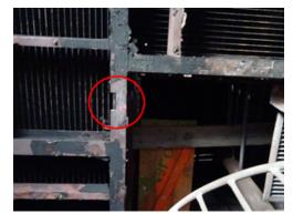
FIGURE 13. Steel sample cut out of floor beam in ZONE 2.
