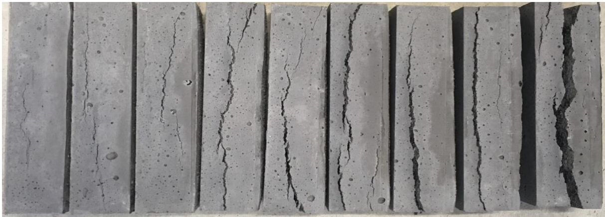
Figure 1 First version of concrete mixture designed in 2019 with waste glass powder from photovoltaic panels.
