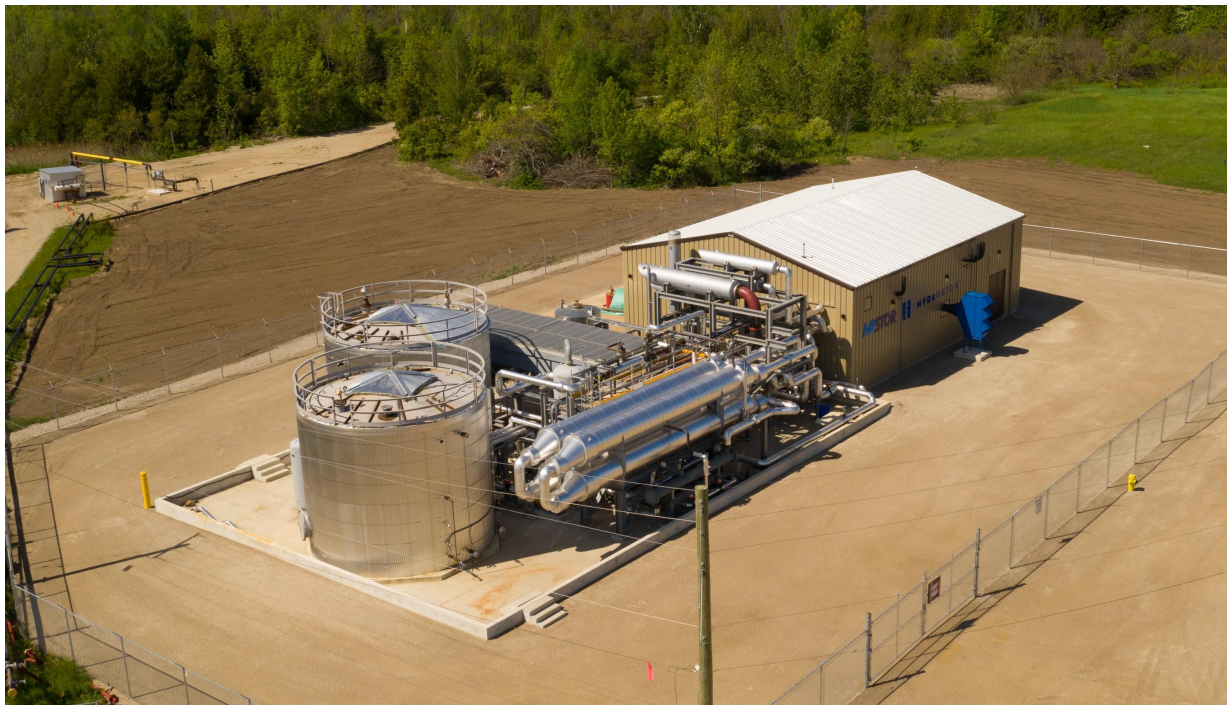
Figure 13 Working Compressed Air Energy Storage (CAES)(13)
