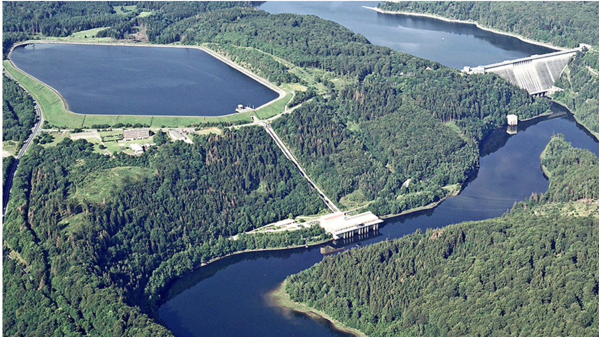
Figure 11 Wendefurth Pumped-storage Power Plant (12)
