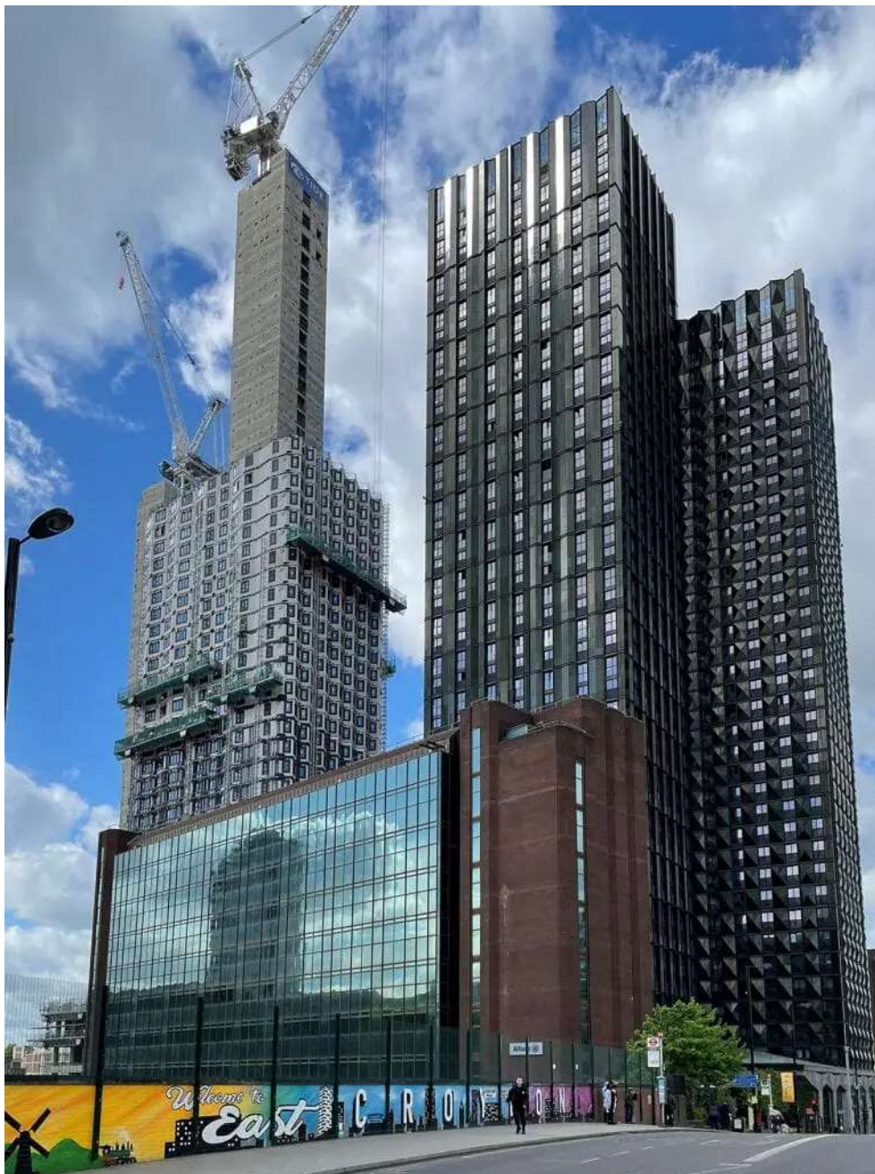
Obr. 2 - 101 George Street a za ní stavba College Road [3]
