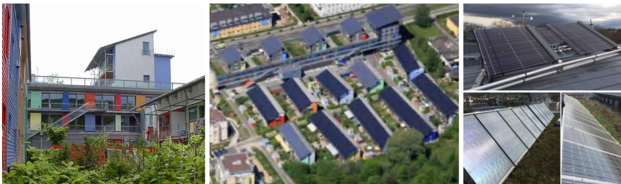
Figure A1.6 Plus-energy residential complex (left and middle) (source: (City of Freiburg, 2008) ); Solar thermal (top right) and Solar Photovoltaic (PV) (bottom right) (source: Bardhyl Rama).
