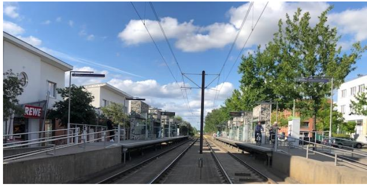
Figure A2.13 View of one of the main Kronsberg tram stop (source: Bardhyl Rama)
