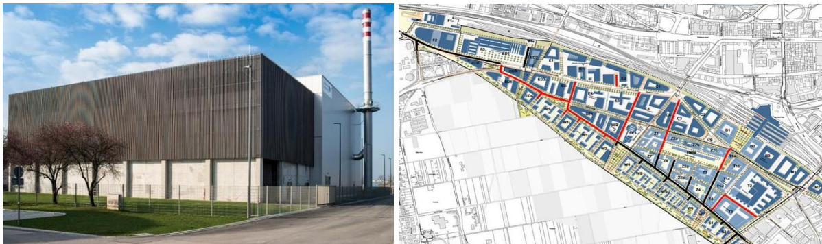
Figure A3.10 Combined Heat and Power (CHP) wood-fired thermal power station (right), district heating network (right) (source: City of Heidelberg)
