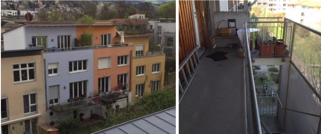
Figure A1.4 Group owner's four-story multi-family houses (left), access to upper unit via outside balcony (right) (source: Bardhyl Rama).
