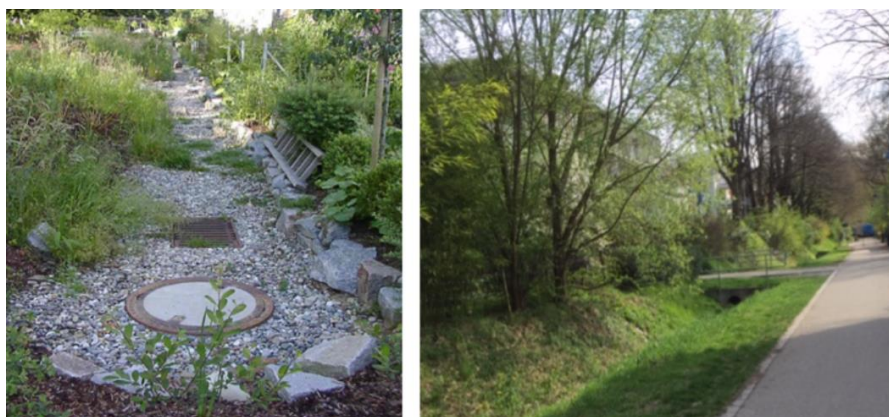
Figure A1.18 Rainwater collection, infiltration area (left) (source: (City of Freiburg, 2008) ); view of functioning open water collection/drainage ditch (source: Bardhyl Rama)
