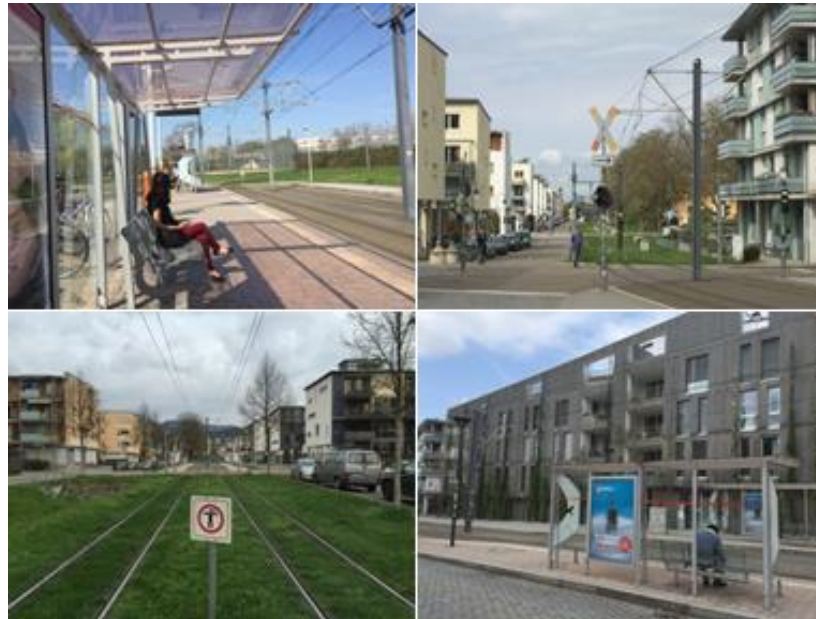
Figure A1.10 View of the tram and bus line and the stops at different points (source: Bardhyl Rama)
