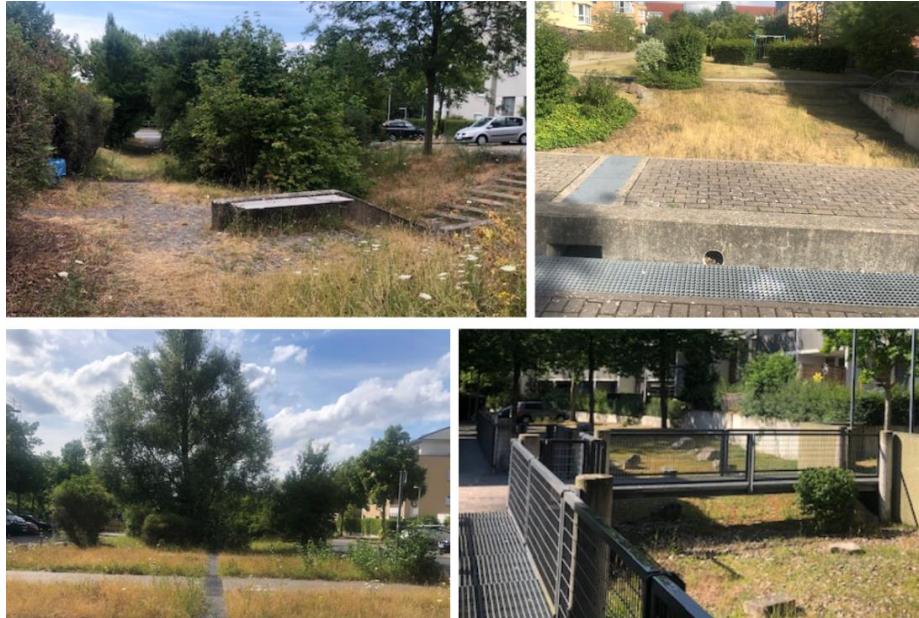
Figure A2.22 Rainwater collection area (source: Bardhyl Rama)
