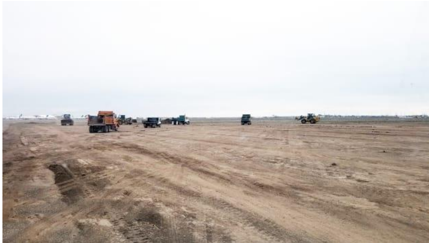
Figure 3 – Roswell Air Center adding more space [22]
