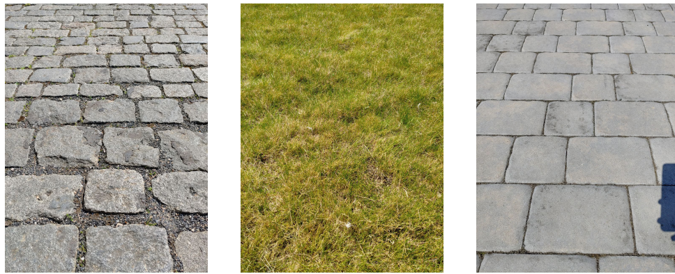
(a) : Sett paving
