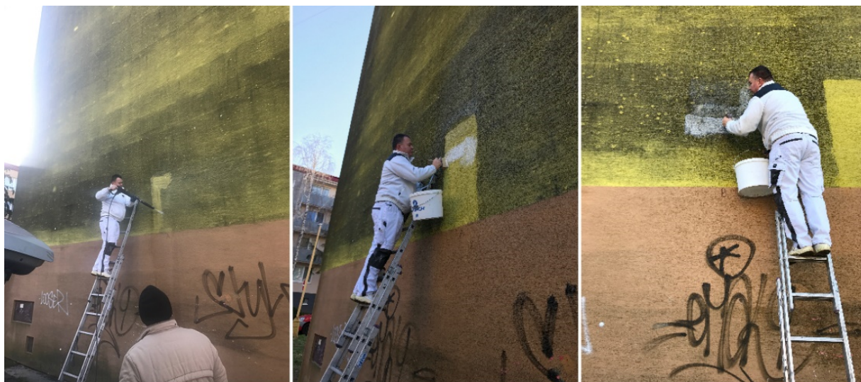
FIGURE 3. Preparation of bottom layer before applying additional insulation.
