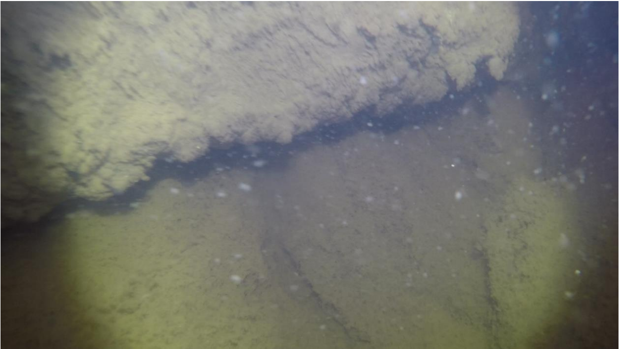
Figure 51 – Camera probe picture of the pillar exit
