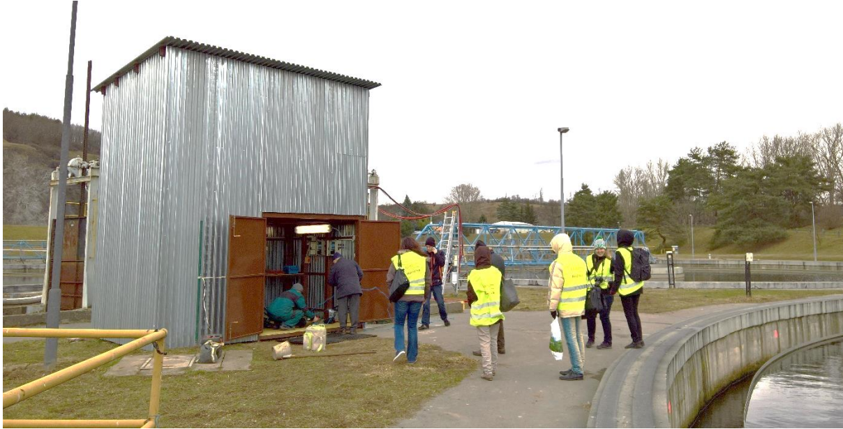
Figure 14 – Field lab built for tests data collection at the CWWTP in Prague
