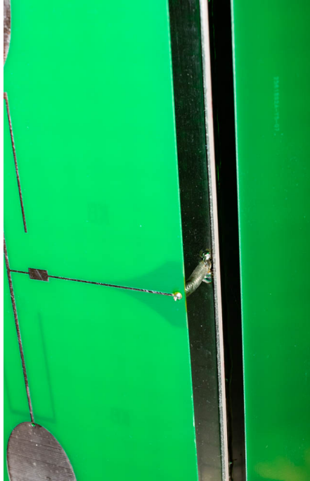
Figure 20: Final connection of the semi-rigid coaxial cable with the sector antenna.
