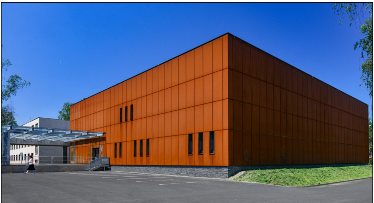
Fig. 38 Depository for the East Bohemian Museum in Pardubice [89]
