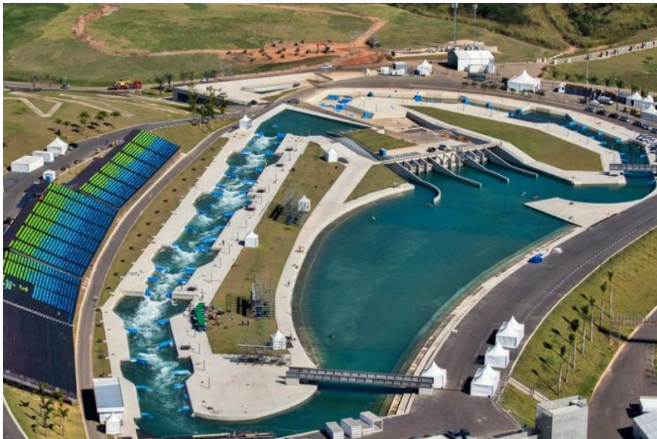
Obrázek 2: konstrukce USD mimo tok se systémem čerpadel (Deodoro Olympic whitewater stadium dostupné na http://rededoesporte.gov.br/en/news/check-out-some-of-the-main-rio-2016-competition-venues-in-detail )
