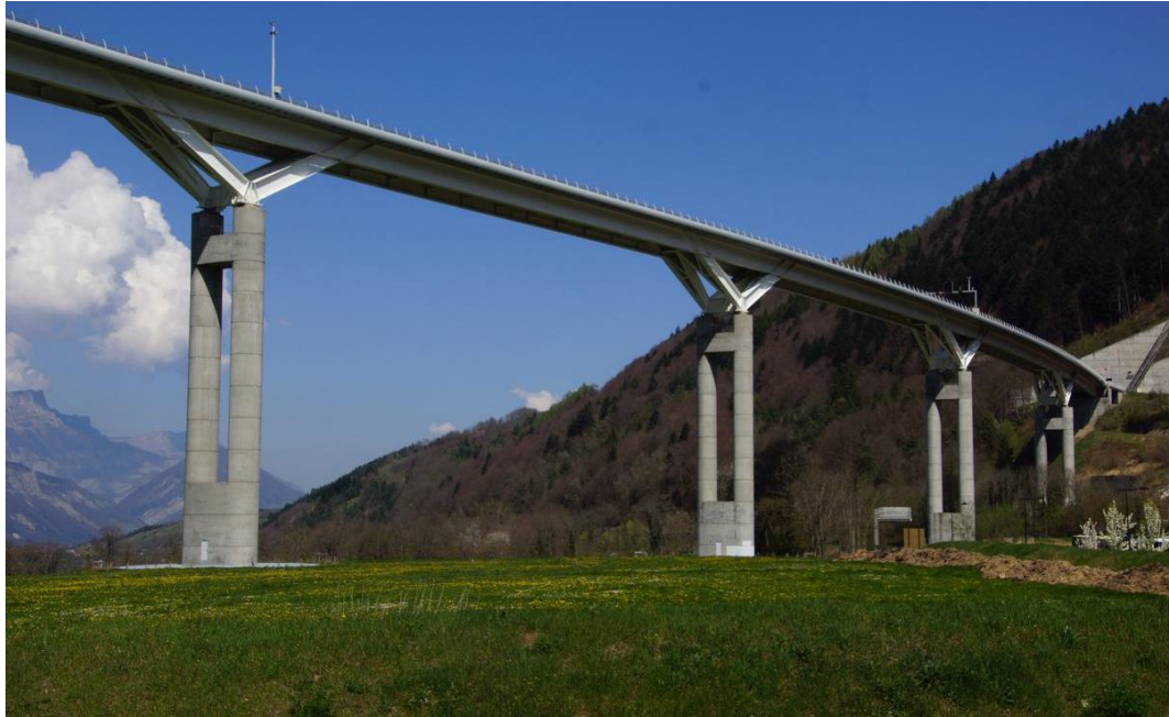
Obr. 25 - Pohled na Monestier viaduct [39]
