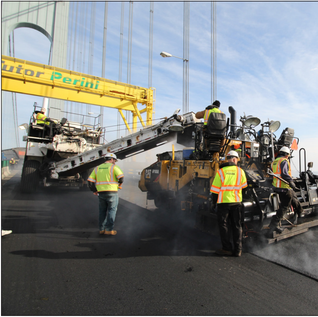
$320M Verrazano-Narrows Bridge Rehabilitation, New York New York Metropolitan Transportation Authority
