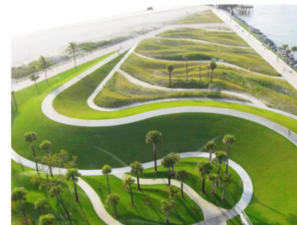
Obrázek 43: South Pointe Park v Miami (William Lane Architects, 2009)
