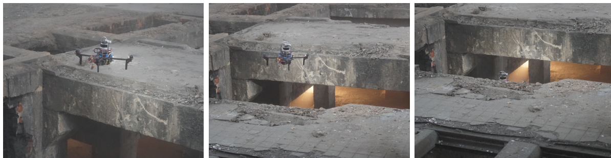
Figure 7.10: The UAV moving through a hole to explore frontiers in the lower level of the brewery.
