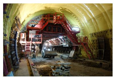
FIGURE 2. The secondary lining construction from in situ cast concrete (photo Hilar).
