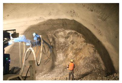
FIGURE 1. The primary lining construction from sprayed concrete (photo Hilar).
