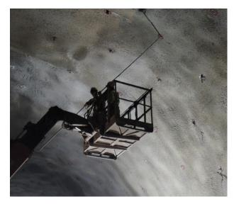
FIGURE 3. Installation of rockbolts (photo Hilar).
